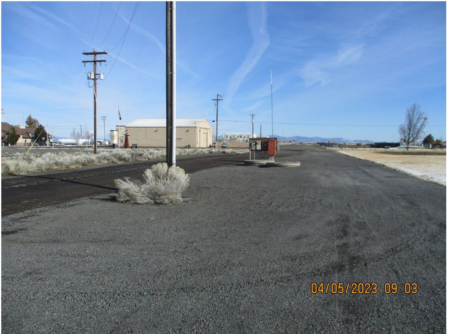
Demers Drive looking north at existing pump station
