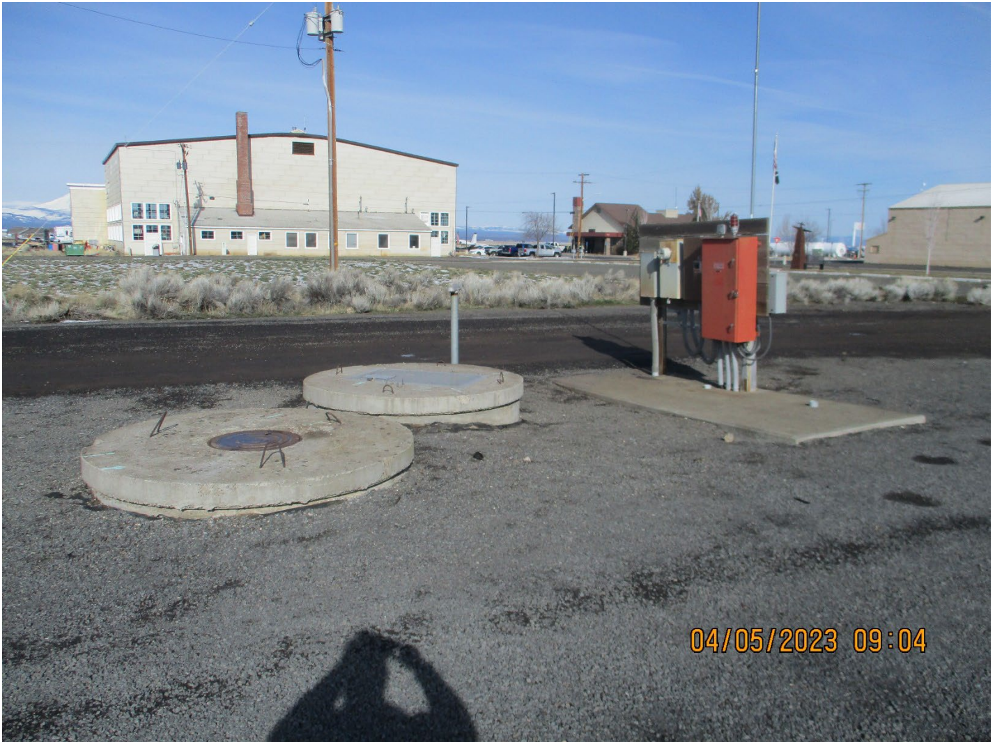
Existing pump station looking west.
