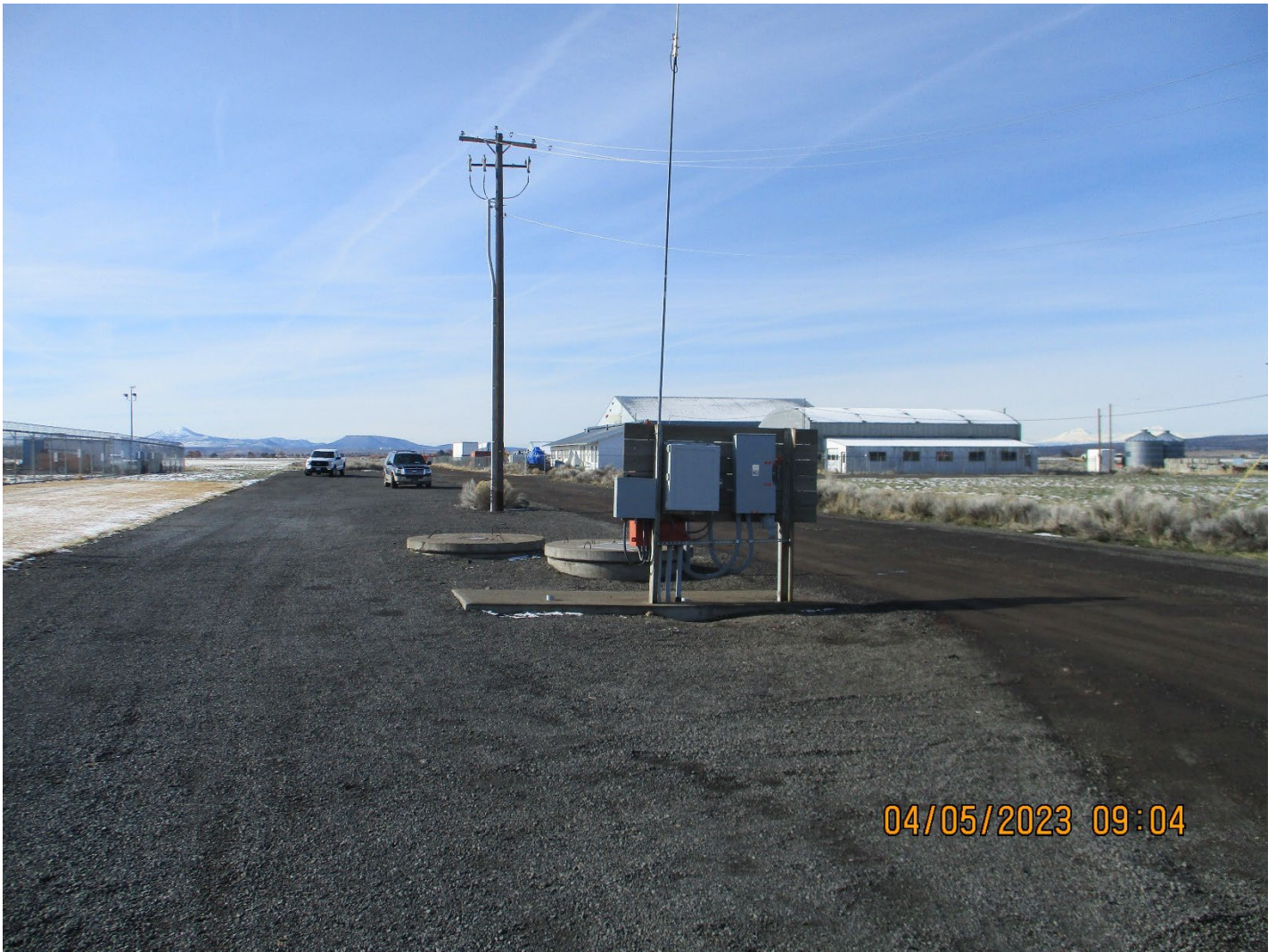
Demers Drive looking south at existing pump station.
